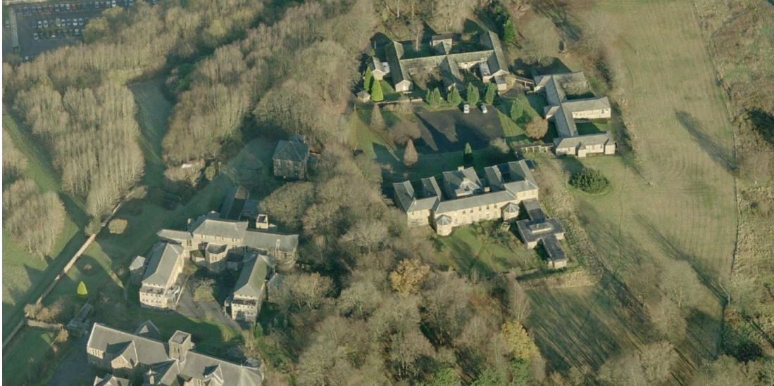
Ancillary housing buildings to the north of the New Block, now demolished for modern residential development ( https://www.bing.com/maps/ )
