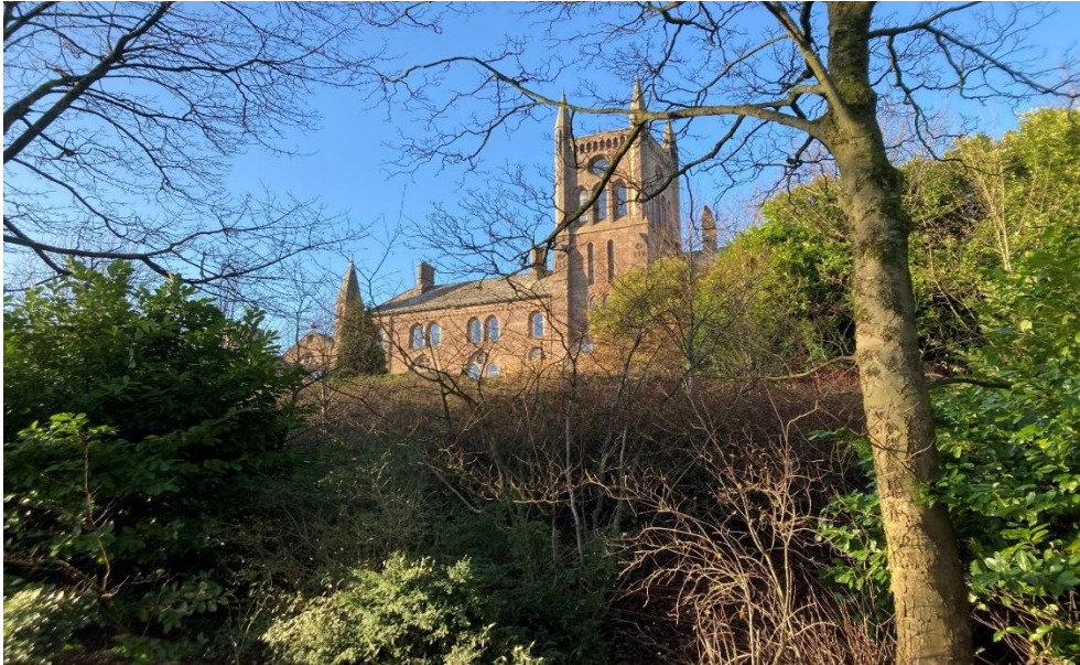
The New Block set within landscaped grounds
