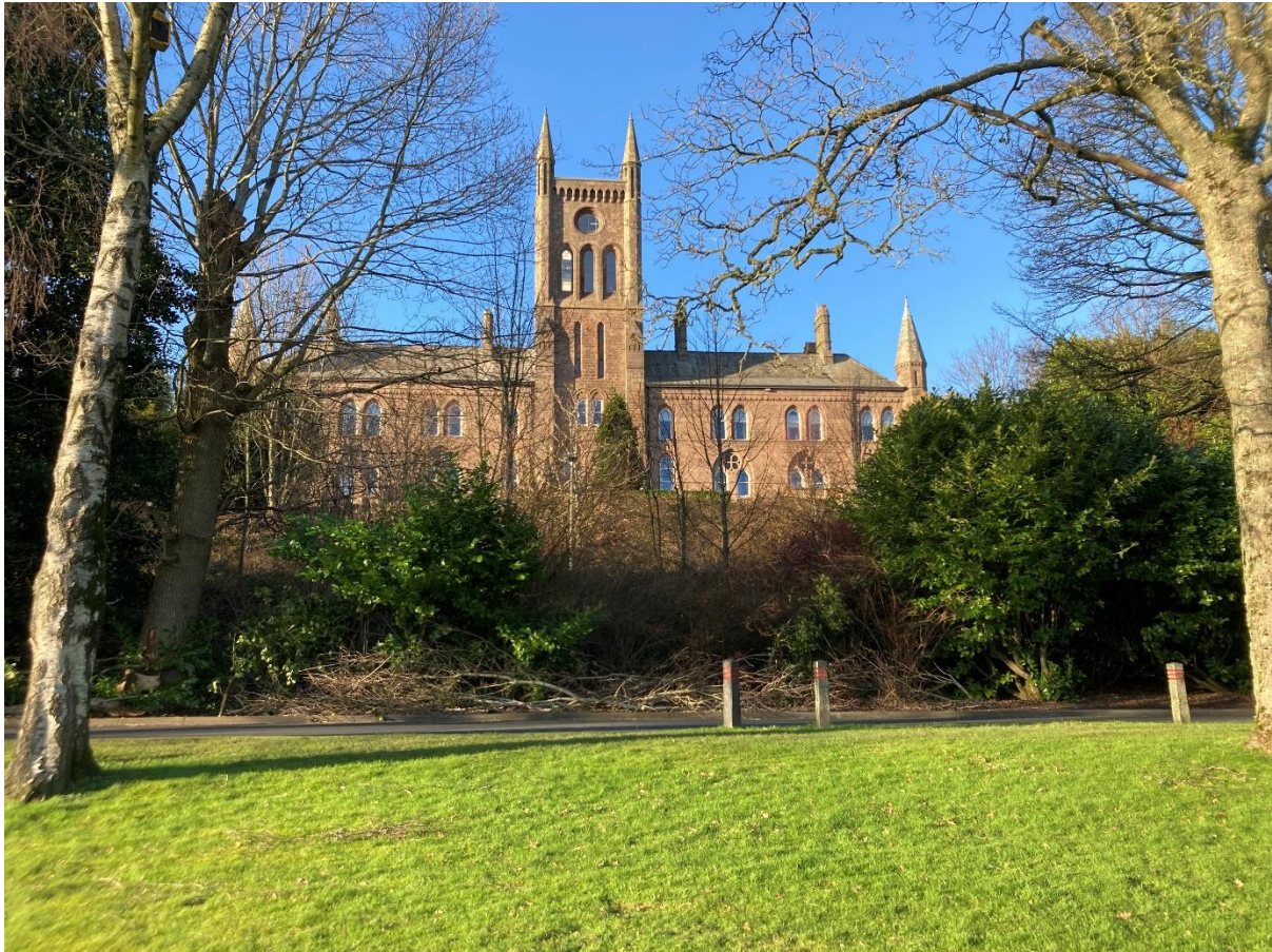
The New Block seen through its wooded setting providing memorable townscape character
