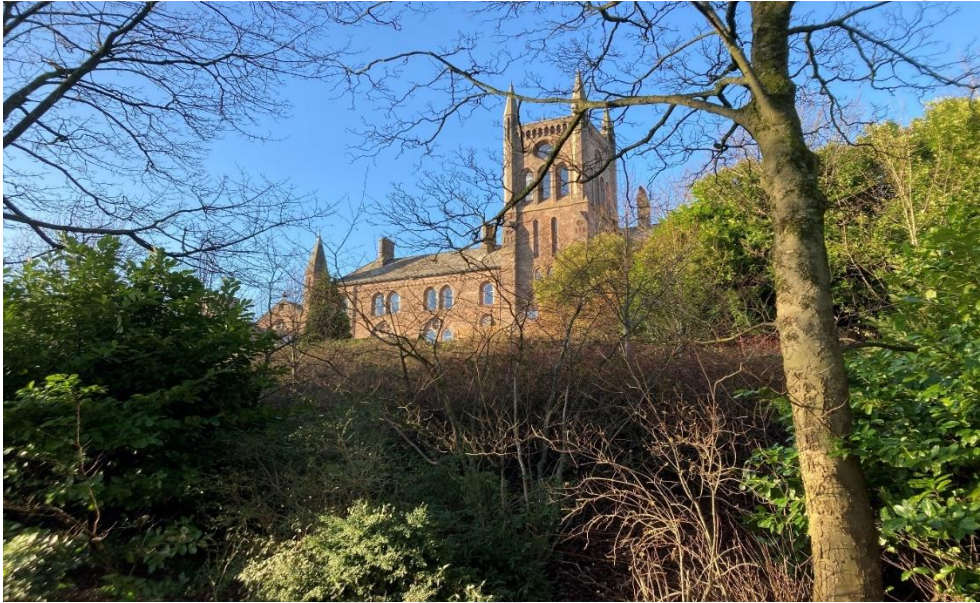
The New Block set within landscaped grounds
