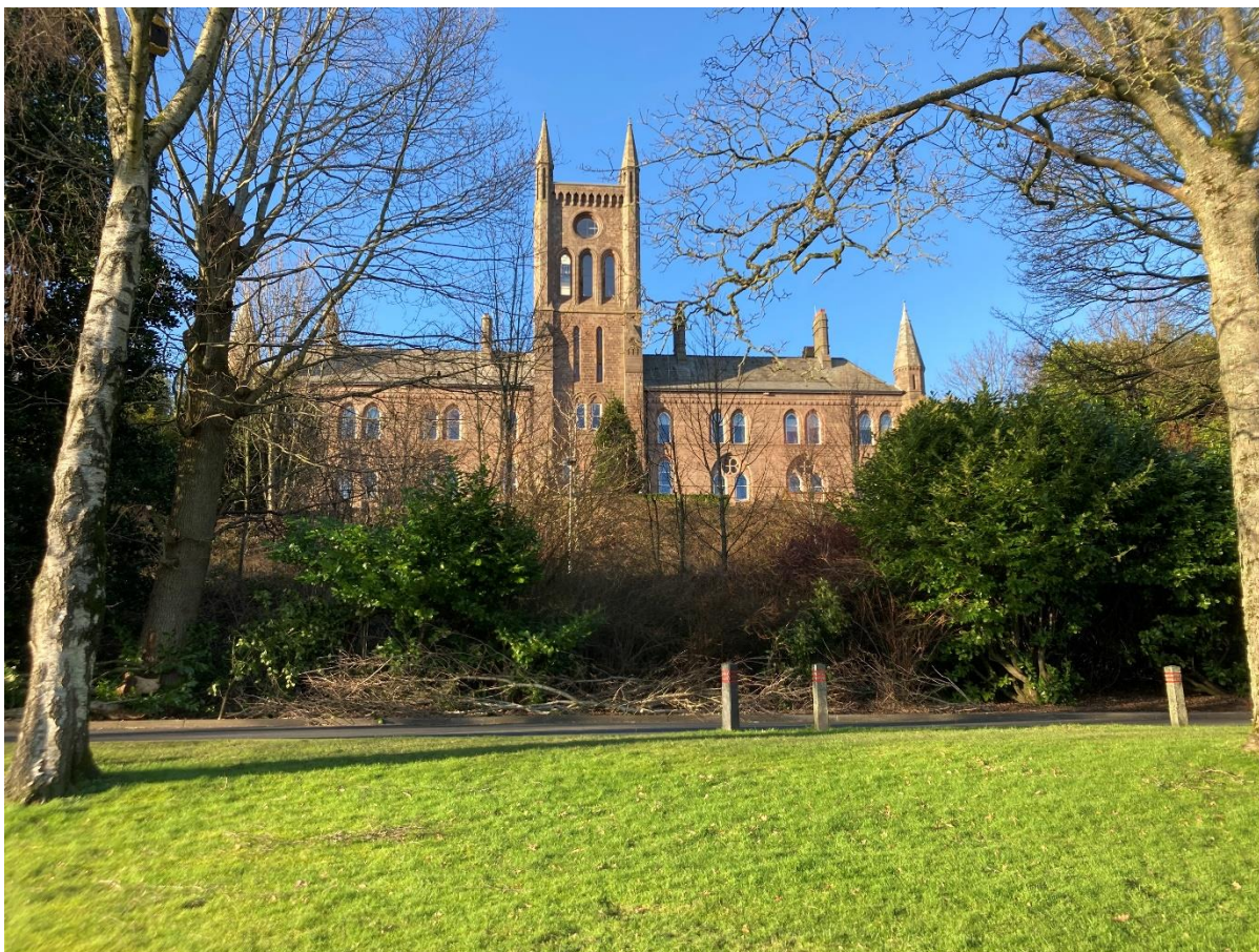
The New Block seen through its wooded setting providing memorable townscape character
